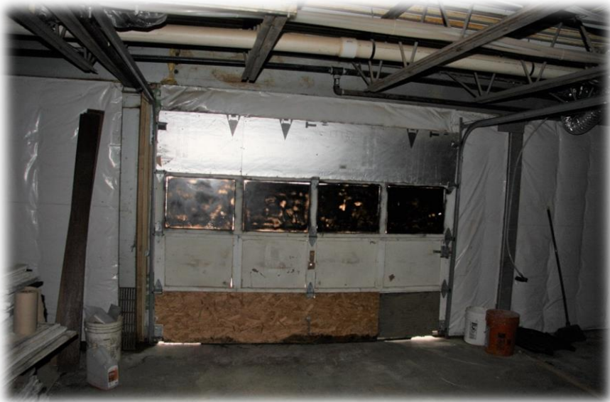
6 FT x 8 FT Overhead door in Basement
